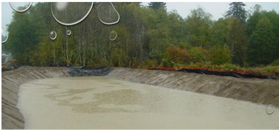
TEMPORARY SEDIMENT POND
